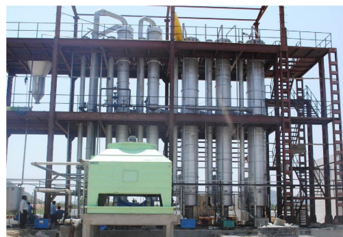
Evaporator being installed at Pertec CETP
