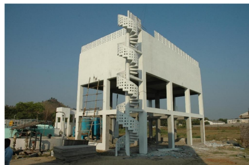
Construction in progress at SIDCO II CETP
